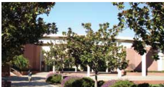
Our new home in the Music and Business Building
