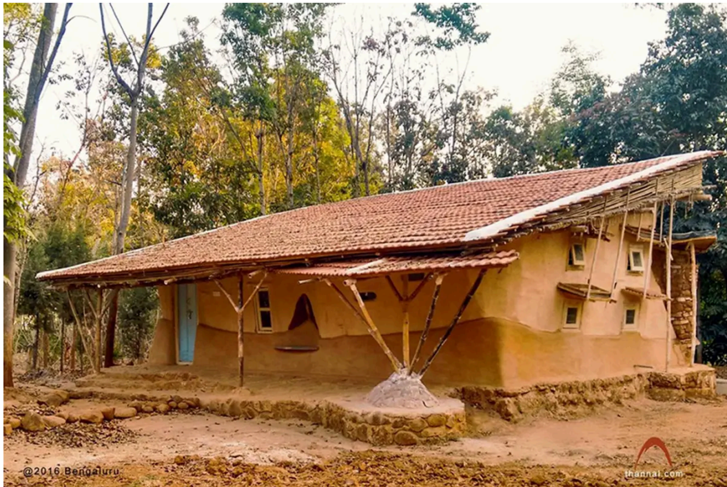
Exterior and interior views of a wattle and daub cottage in Bengaluru, India by natural building pioneer firm Thannai
